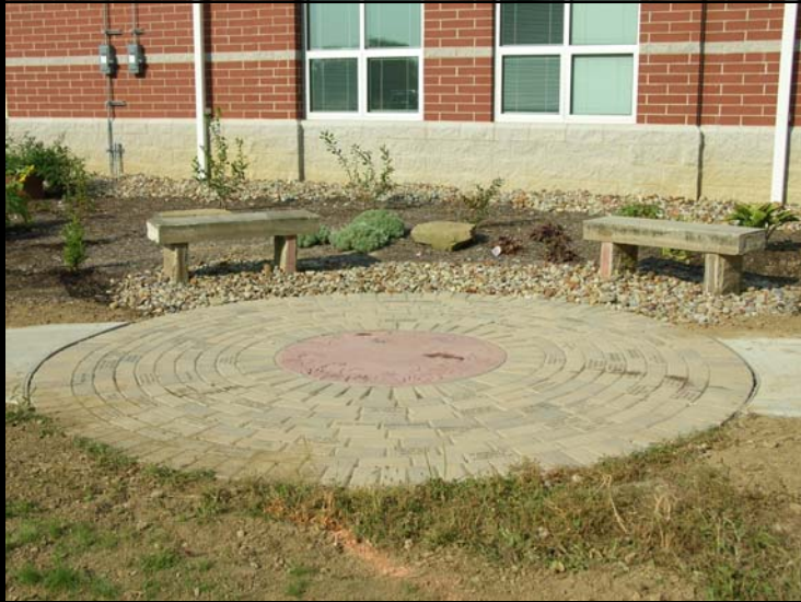
Recycled Construction Materials were used from the demolished Sterling and Burbank Elementary Schools to create benches, etc.
